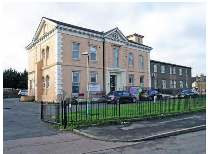
The former council offices at Northfleet. In the basement of this and under the car park to the rear was Northfleet's control centre
